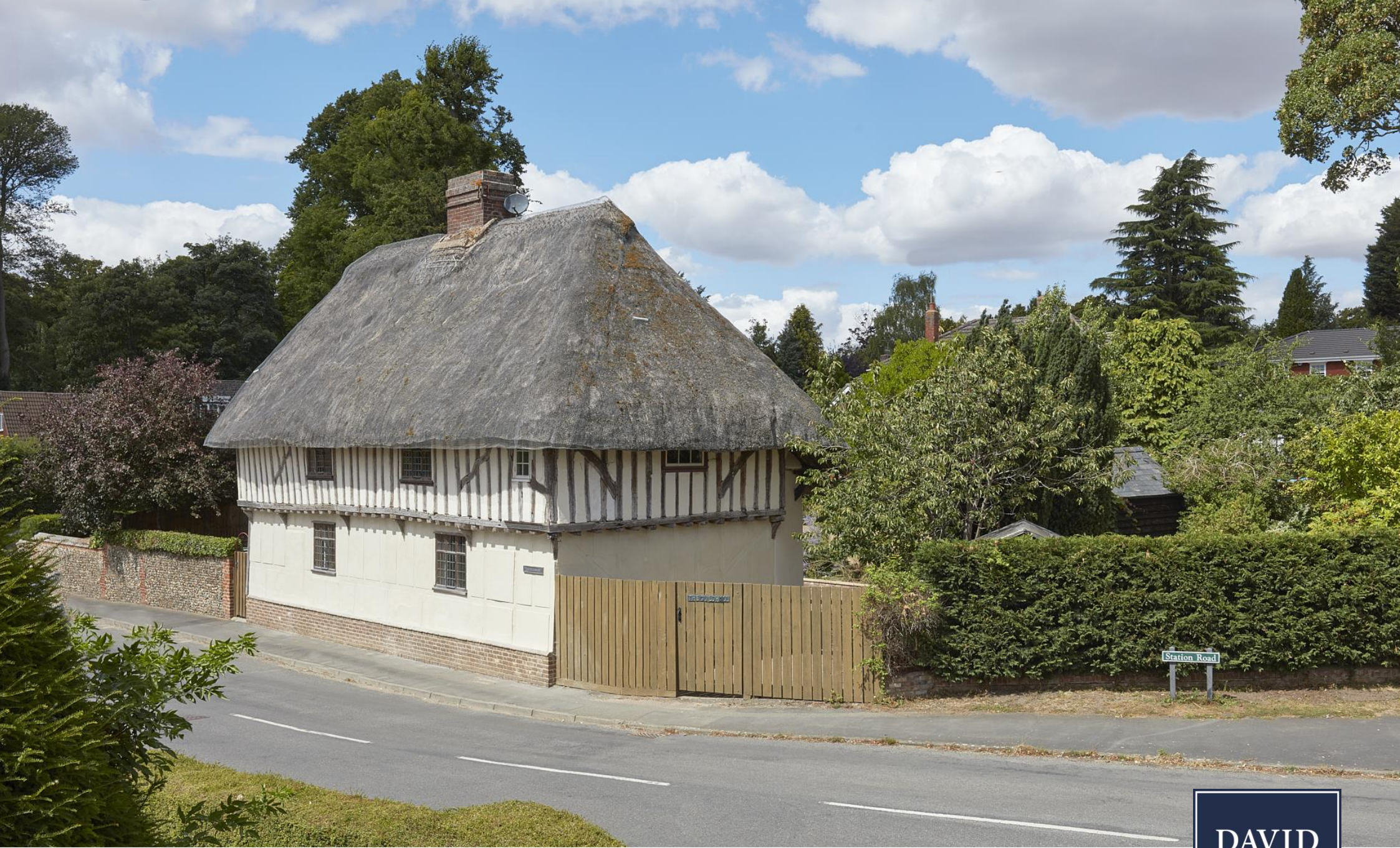
The Guildhall 2-4 Station Road, Dullingham
