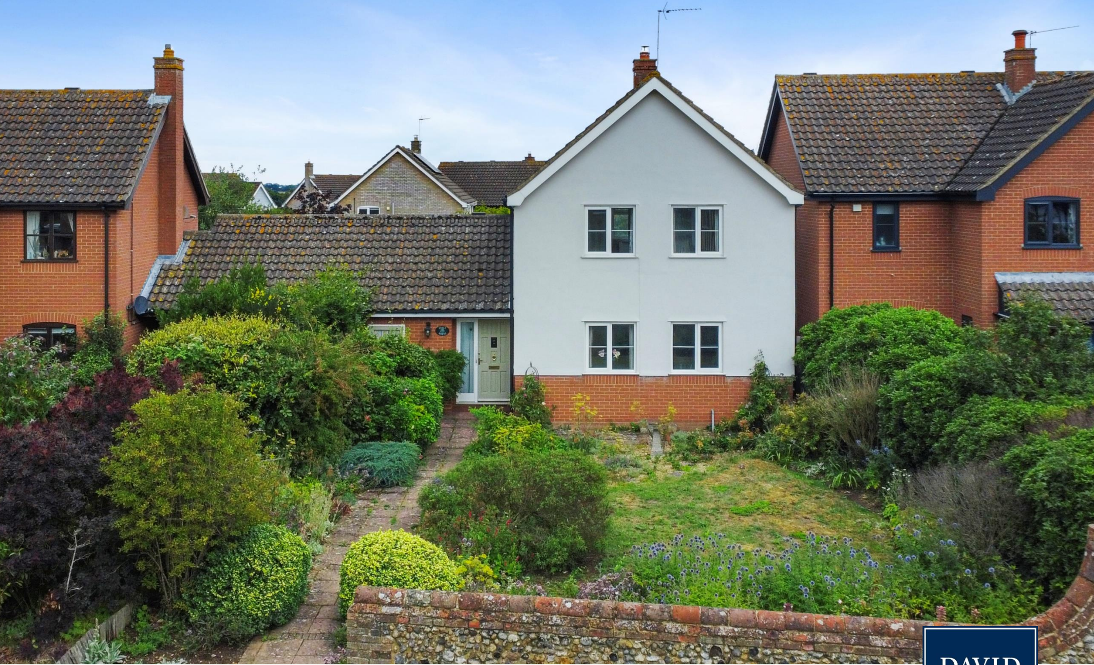
Edale House Woolpit, Suffolk
