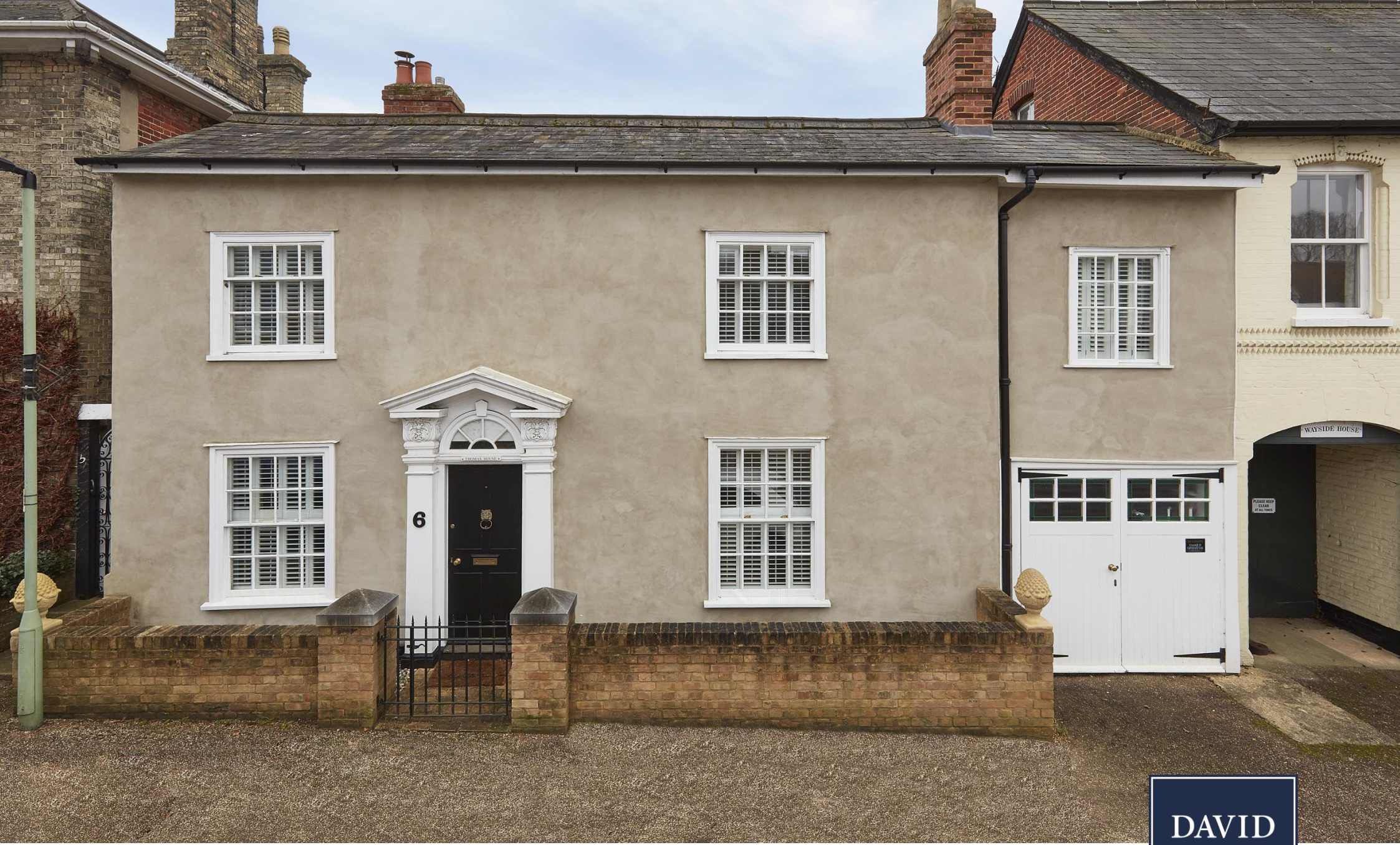
Thomas House 6 Nethergate Street, Clare, Suffolk
